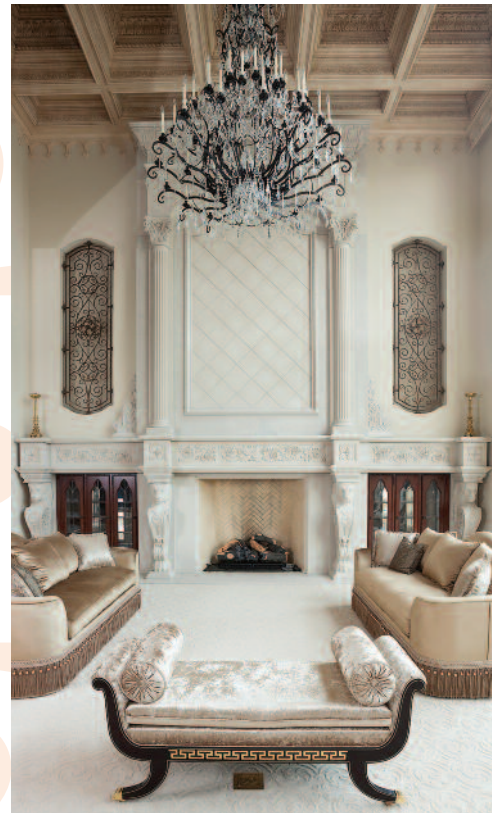
HAND-CARVED INDIANA CUT LIMESTONE. FRISCH MASONRY RECOMMENDED MAKING THE PIECES OF THE FIREPLACE AS LARGE AS POSSIBLE IN ORDER TO ELIMINATE JOINTS.
