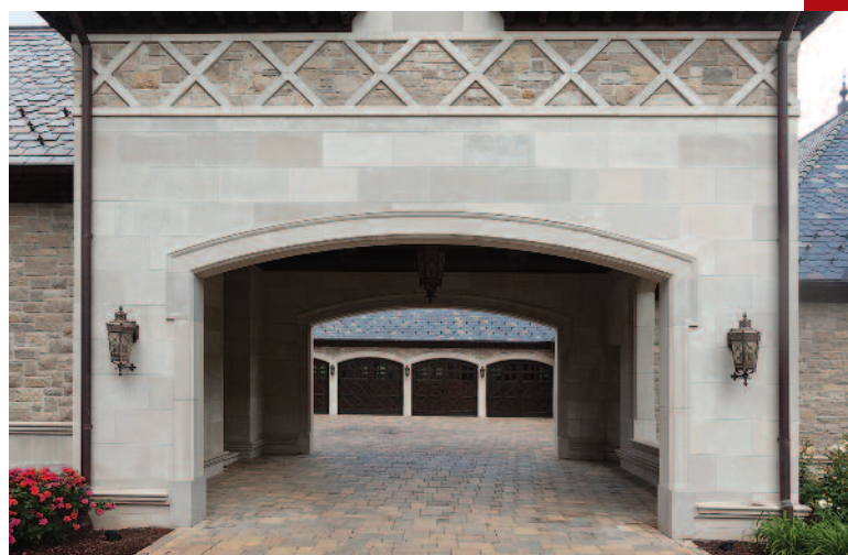
ON THE CARPORT ENTRYWAY, A CUT LIMESTONE ARCH IS HELD IN-PLACE BY STAINLESS STEEL ANCHORS WELDED TO A STEEL BEAM. NOTE THE DECORATIVE X-BAND ABOVE.
